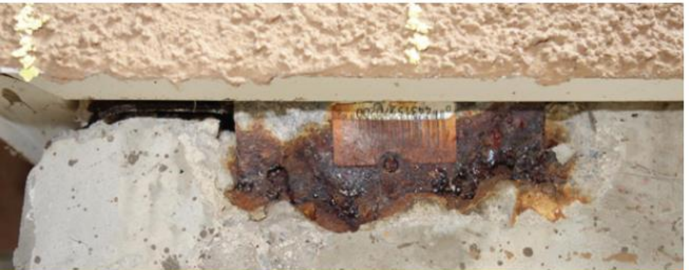
Corroded Anchor Visible Below Cladding
